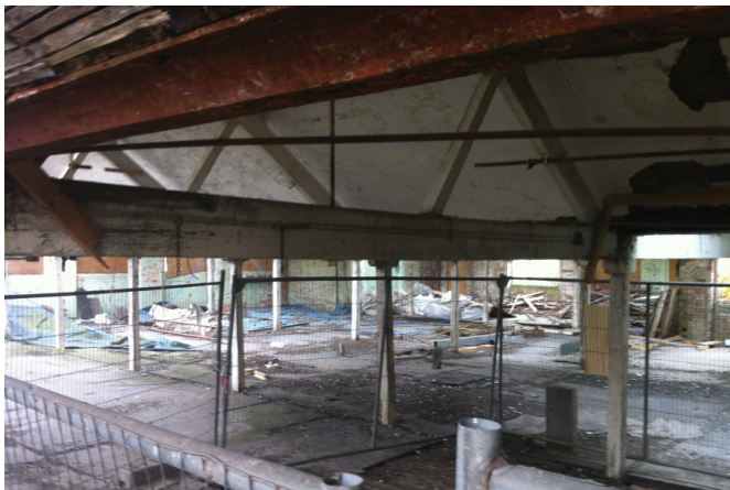
Building C - First Floor (Areas of collapsed Floor)
