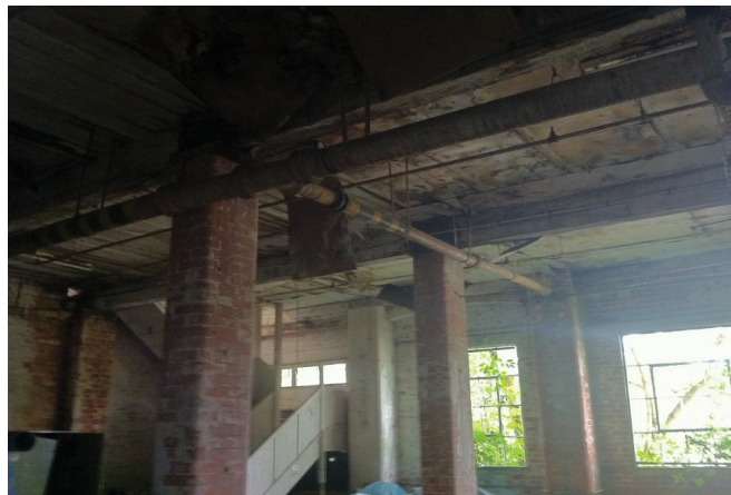
Building C - Ground Floor (Masonry Piers supporting timber beams & floor)
