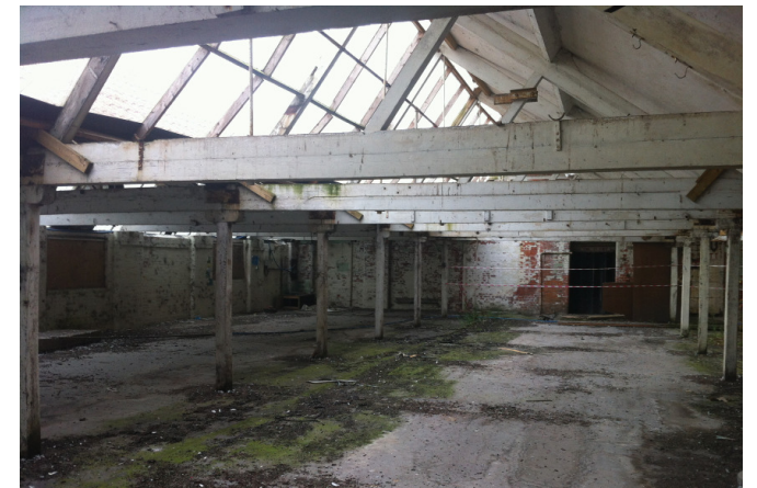
Building C - First Floor (Timber Trusses and 'missing' north light glazing)
