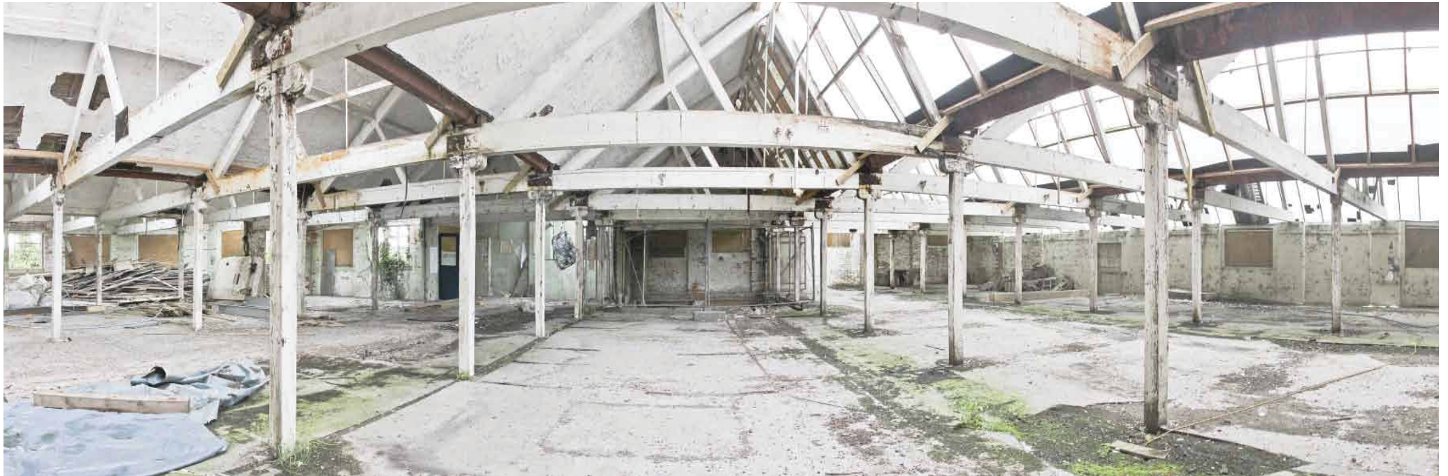
Building C - First Floor (Saw-tooth roof open to the elements above)
